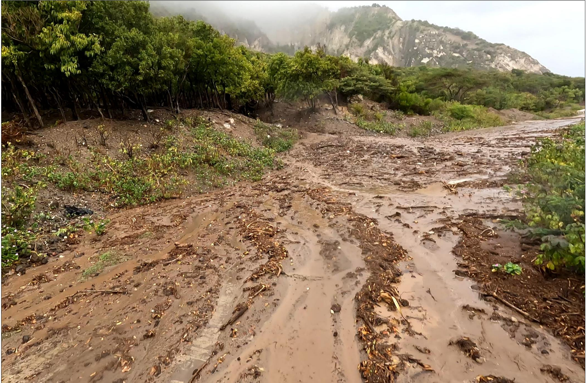
Photo 17 – Weg naar White Wall × Active gully intersections after major flooding 7-1-2023
