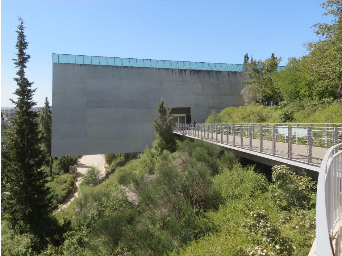
Fig. V: The Holocaust History Museum and the Bridge to a Vanished World leading to its entrance © Author
