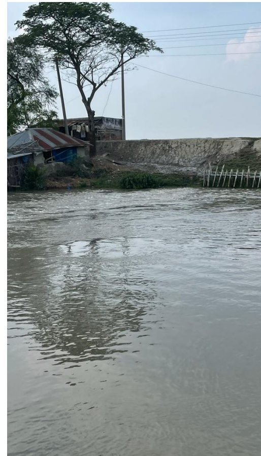
Figure 5b: Switch gate from below
