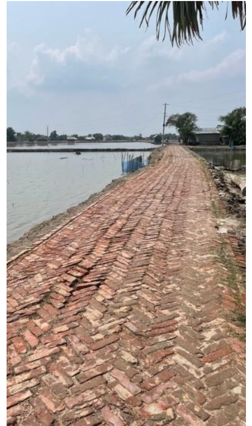
Figure 13: Roads in the shrimp area
