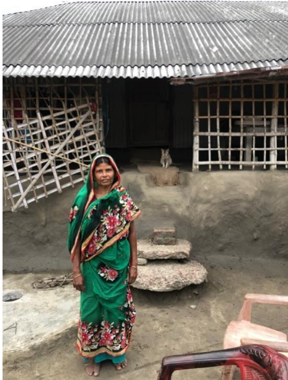
Photograph 11: Elevation of the foundation of her house
