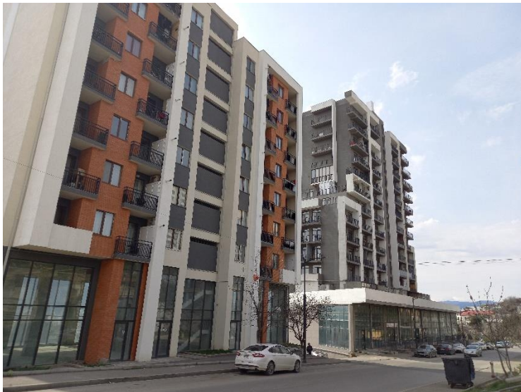
Figure 39 - A new Apartment Block in Vazisubani
