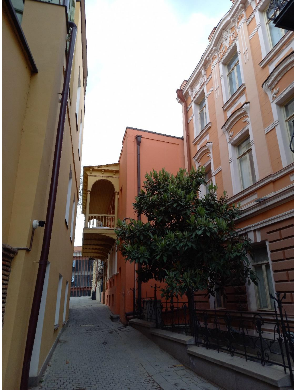
Figure 49 - Newly Refurbished Houses close to Gudashvili Square
