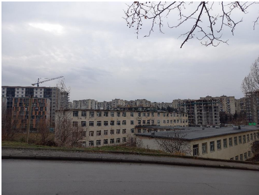
Figure 2 - Housing Estates in Gldani
