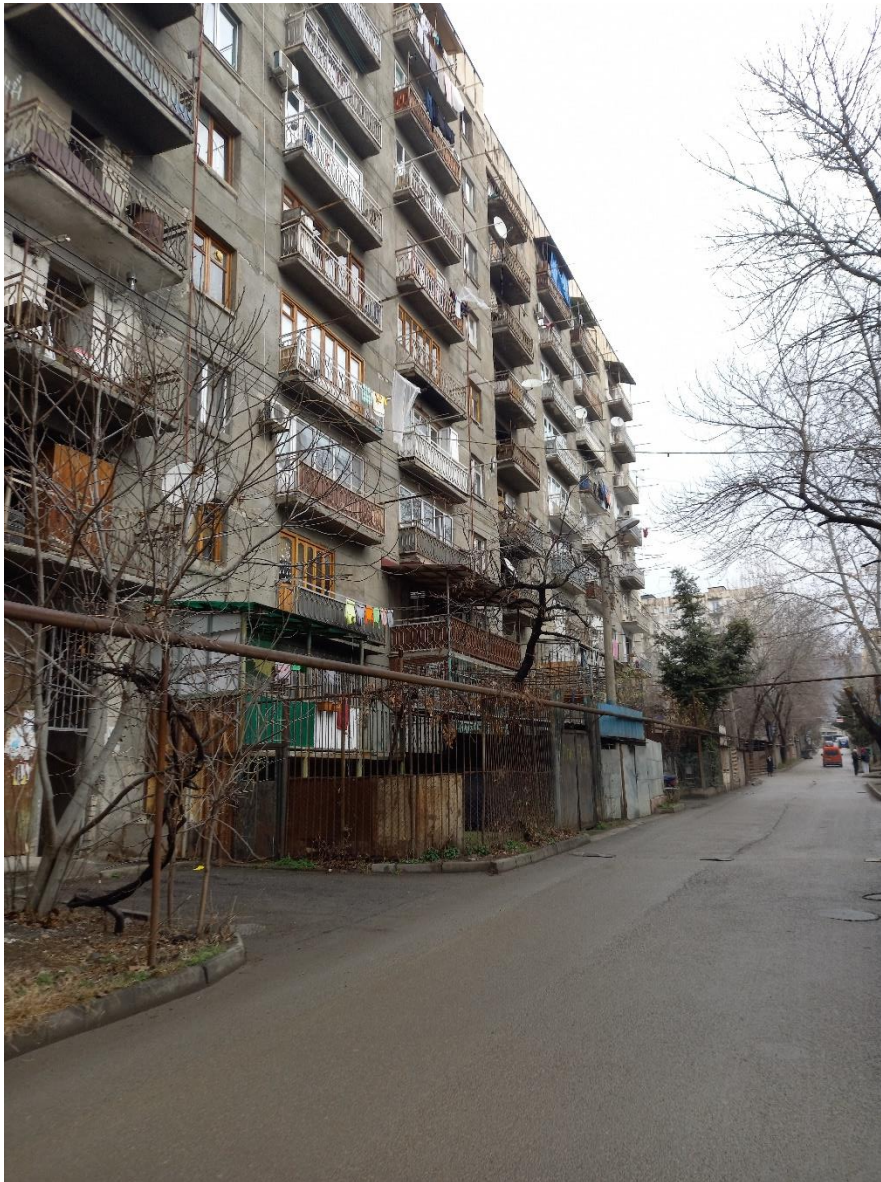
Figure 71 - An Apartment Block in Gldani
