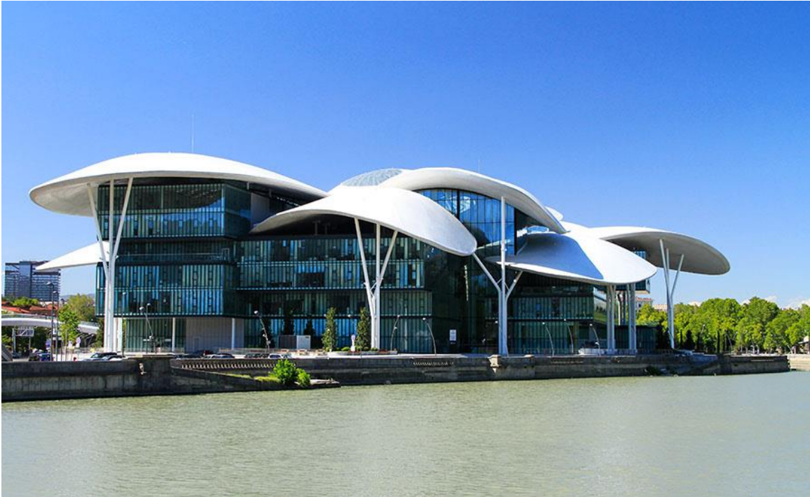
Figure 62 - Public Service Hall next to the Mtkvari River
