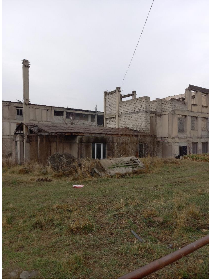
Figure 4 - Abandoned Industrial Buildings in Gldani
