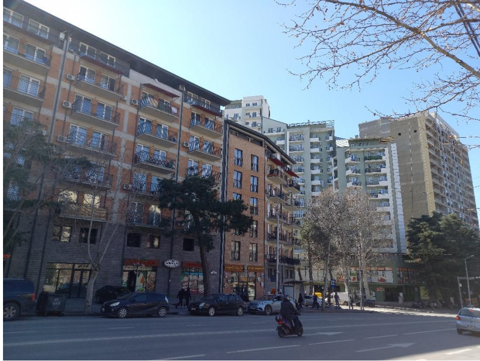
Figure 1 - A New Housing Development in Didube
