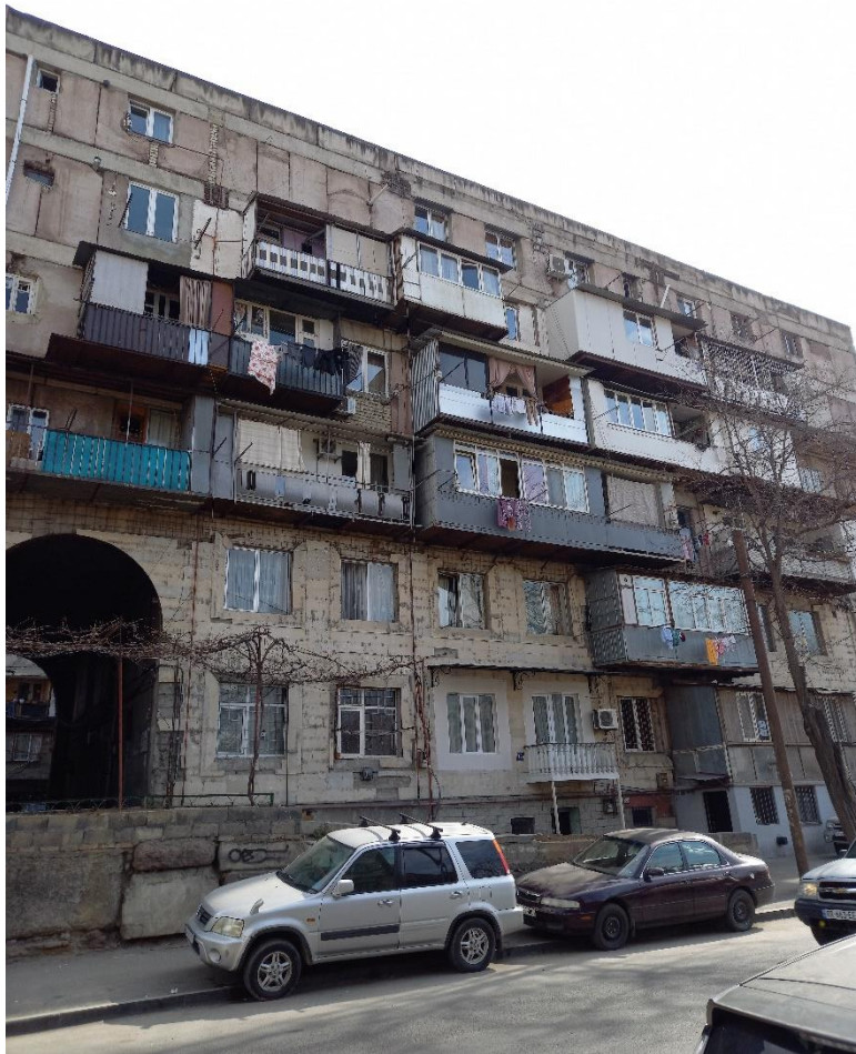
Figure 33 - An apartment block in Nadzaladevi
