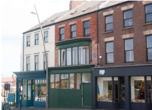
Fig. 20: Pop Recs before after renovation (Liebenrood, 2022)
