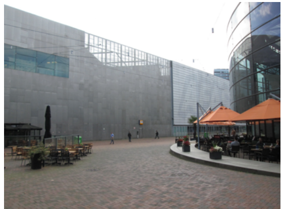
Figure 26: Metal building at the west side station area. Source: Respondent Ed.
