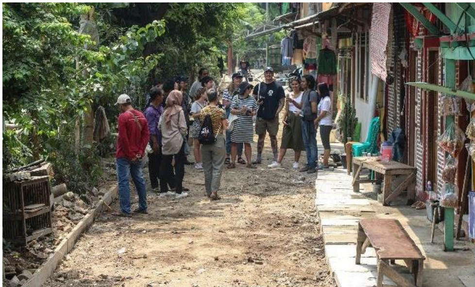
Picture 13: Road construction by the community (2) (source: Gugun, 2015)
