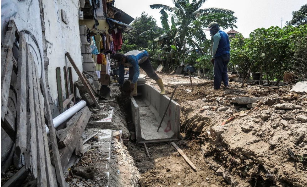
Picture 15: Septic tanks construction process (source: Gugun, 2016)
