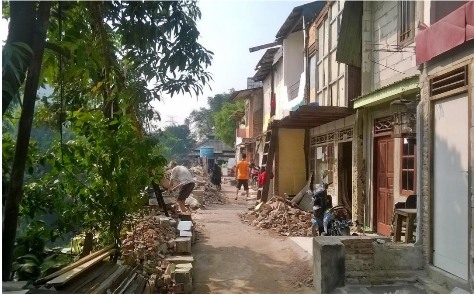
Picture 12: Road construction by the community (1) (source: Gugun, 2015)
