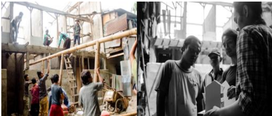
Picture 16: Sample House construction process (source: Gugun, 2015)
