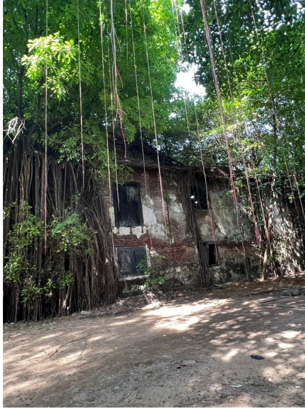
Picture 1: Inside the old historical building (source: author, 2023)
