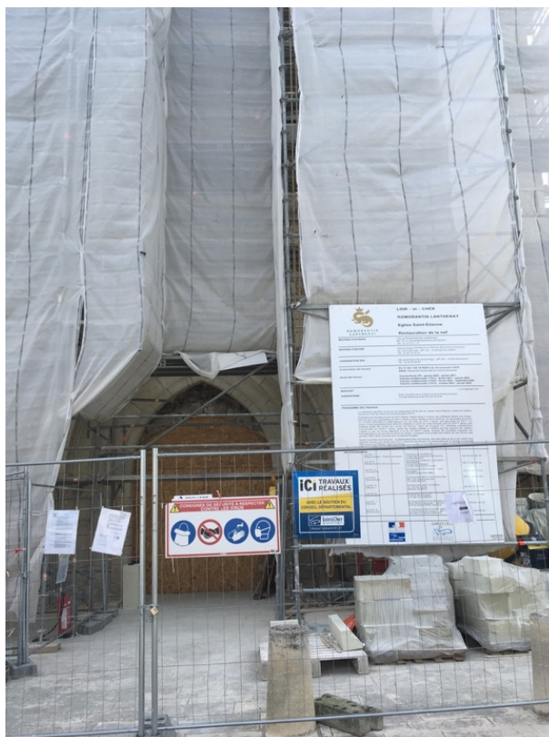
Figure 51 (source: my own): façade of the Saint-Etienne Church in April 2023
