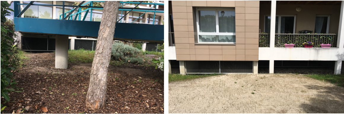
Figure 36-37 (source: my own): metal gratings of the car park at Domitys
