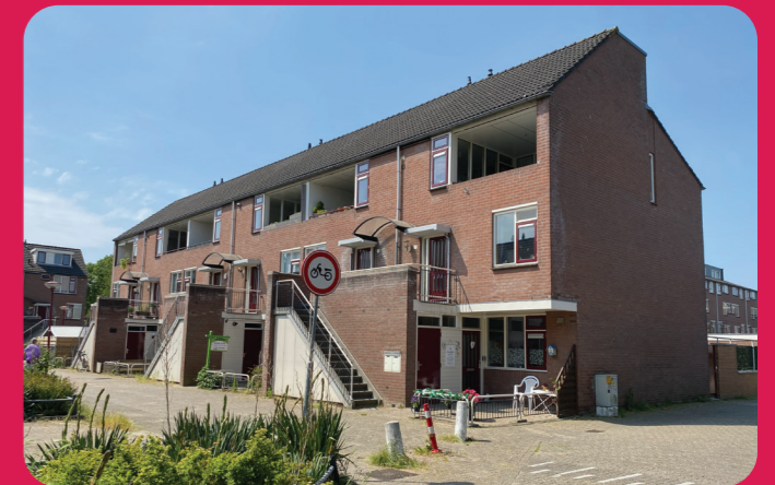
Figure 4.52: Apartments in Nieuwegein that are only accessible through stairs. Makes it impossible for persons with disabilities to live here.
