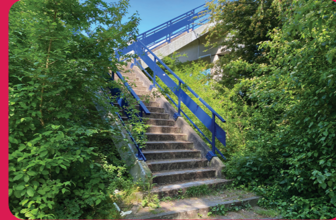
Figure 4.47: Bus stop in Purmerend that is not accessible for persons with disabilities or people with mobility issues.
