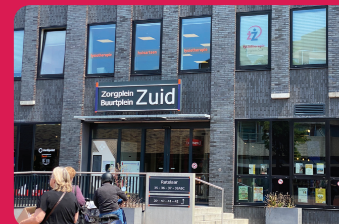
Figure 4.23: Redeveloped healthcare centre in Nieuwegein, Zandveld.
