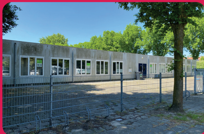
Figure 4.14: Abandoned elementary school in Purmerend, Purmer-Zuid.
