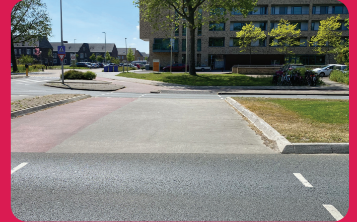
Figure 4.48: Pedestrian crossing in Purmerend that provides median strip to make it easier to cross the road. Especially helpful for people that walk at a slower pace.
