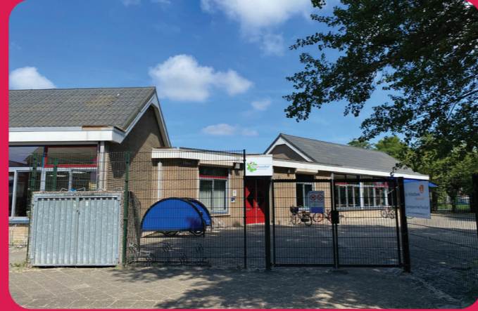
Figure 4.11: Different functions in a school building in Purmerend. Unused classrooms are filled with functions such as a library and a childcare centre.
