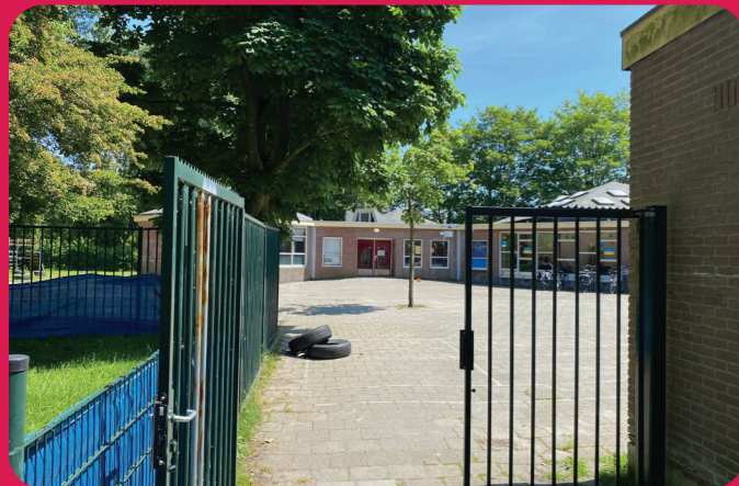
Figure 4.12: Former elementary school in Purmerend that is now being used as housing for Ukrainian refugees.
