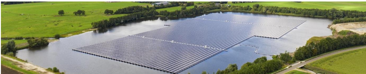
Figure E1: FPV system located in Beilen (Drents Overrijsselse Delta, 2022)
