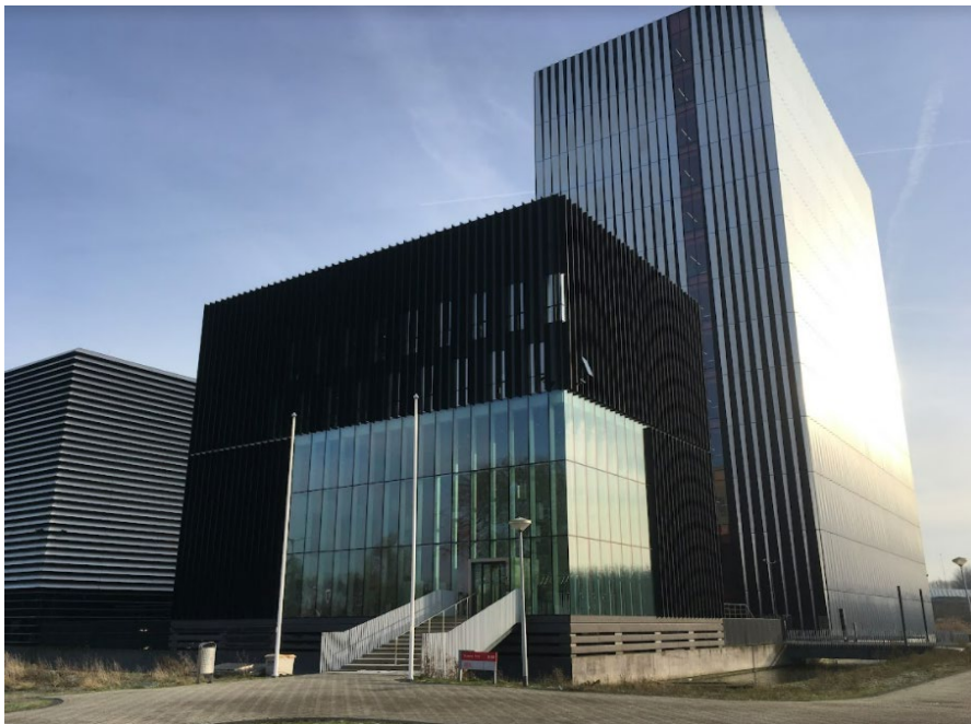
Figure 2. Equinix Data Center Science Park, Amsterdam
