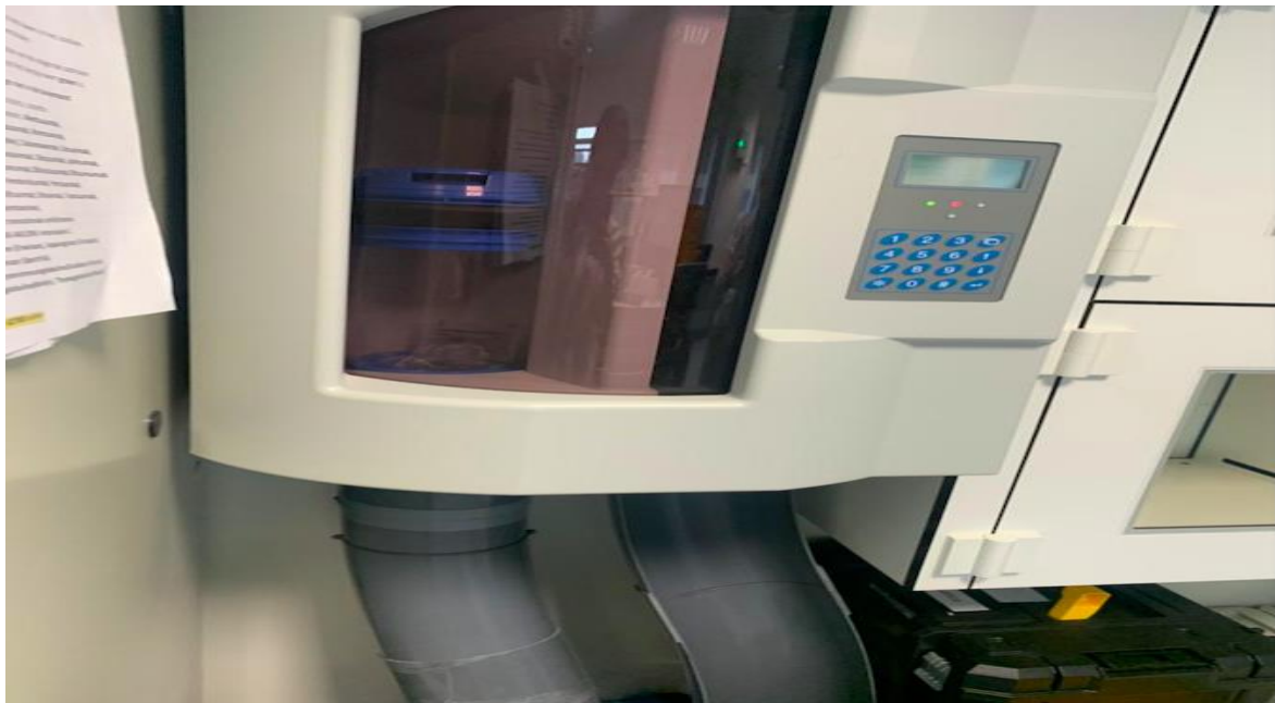
Figure1: This figure shows a picture of Pneumatic Tube Transportation (PTT) in Amsterdam Academic Medical Centre (Amsterdam AMC).
