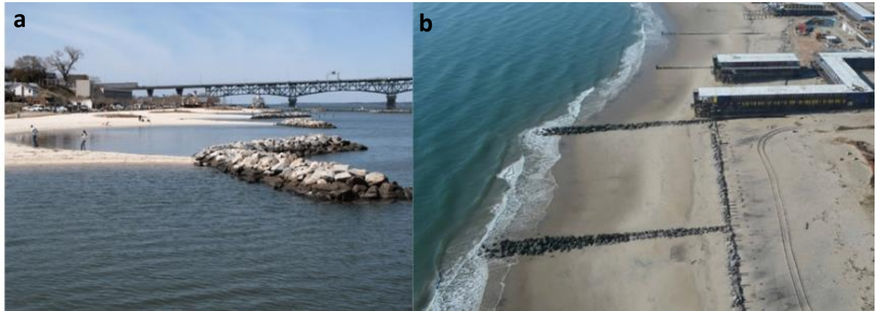
Figure 2. Two examples of coastal protection by the integration of hard structures. a) breakwater that stimulates sediment accretion at Colonial National Historic Park, Virginia (Steve Simons, 2012). b) groin structure along the coast of New Jersey (NPS photo, n.d.)
