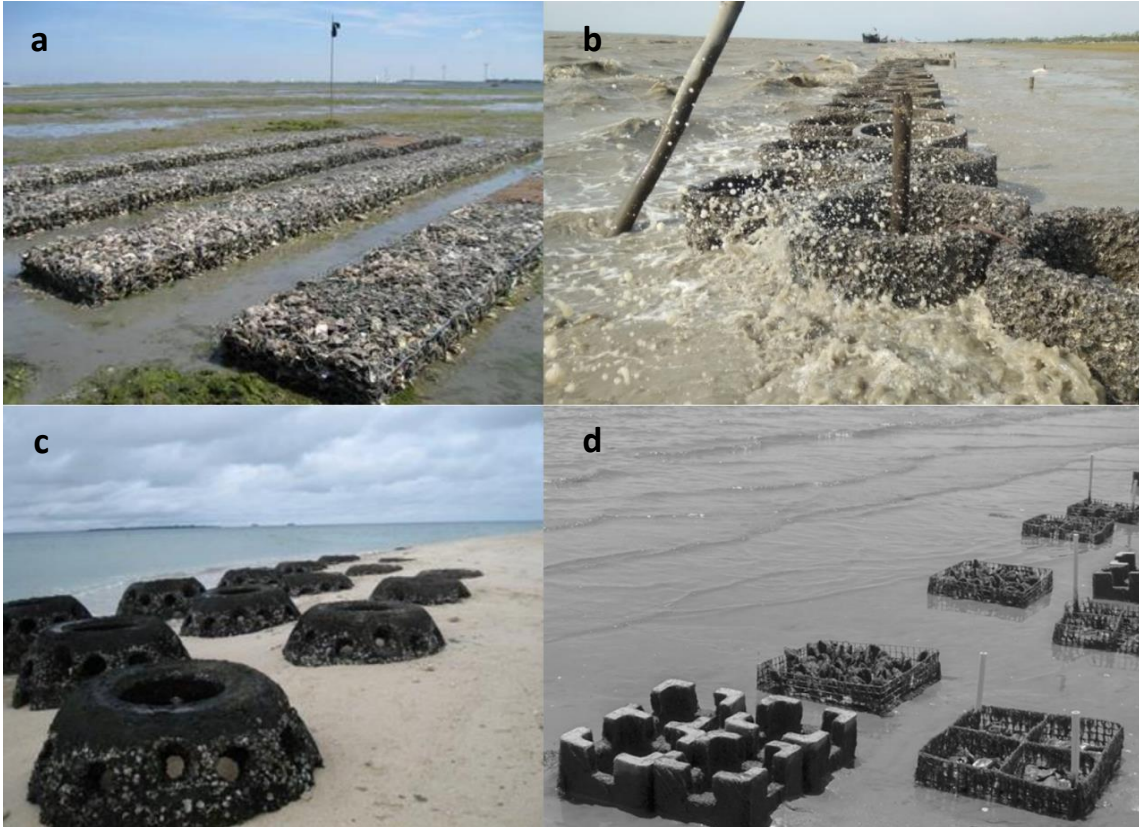
Figure 4. Artificial oyster reefs are used in different forms and configurations. a) gabions filled with empty oyster shells at the Eastern Scheldt, The Netherlands (Oyster Reefs, 2009). b) concrete rings used to protect salt marshes at an island of Bangladesh (Chowdhury et al., 2019). c) reefballs at Sabah, Malaysia (Saleh et al., 2018). d) oyster castles at Chesapeake Bay, North of United States (Theuerkauf et al., 2015).
