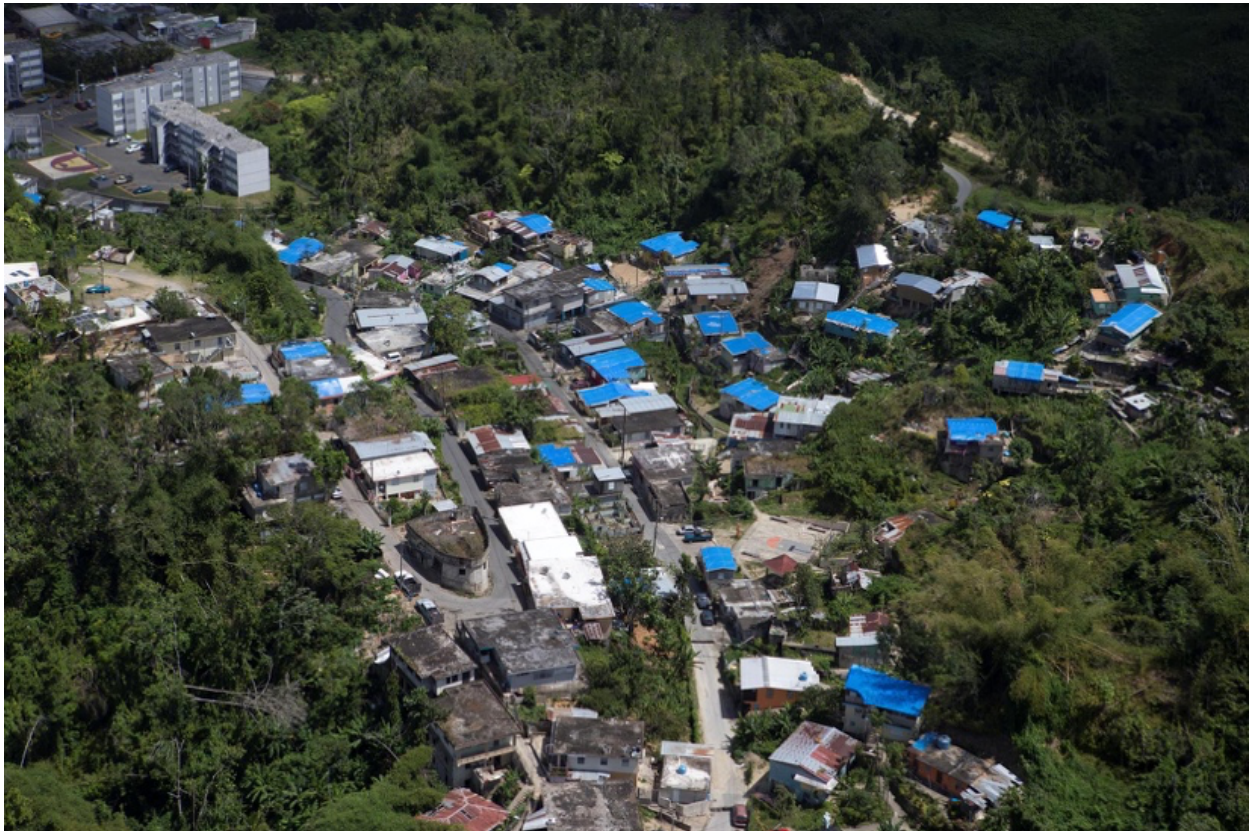
Figure 7. Photo of Blue Tarps on 3,646 Structures in P.R. 5 Years After Hurricane Maria (Kuilan, 2022)
