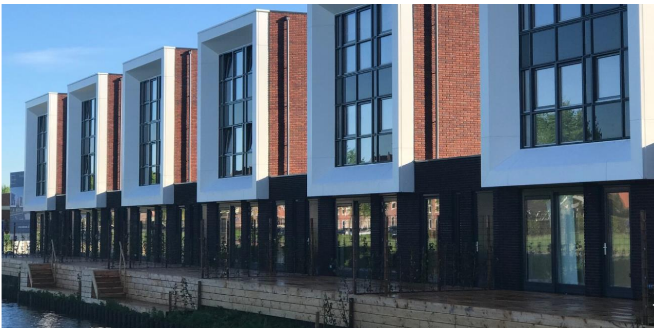
Figure 31 Finished TFC dwellings produced by VolkerWessels in their 'Morgen Wonen' factory Source: MorgenWonen (n.d.)
