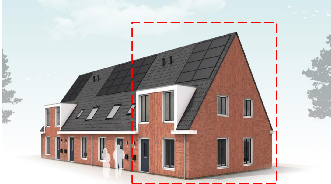
Figure 11 Two storey dwelling with pointed roof that serves as case study dwelling for this study. It has been constructed with the prefab CMC approach and is expected to be produced with the TFC approach until 2030.
