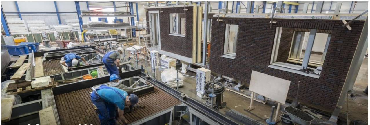
Figure 30 Inside the VolkerWessels TFC factory Morgen Wonen
