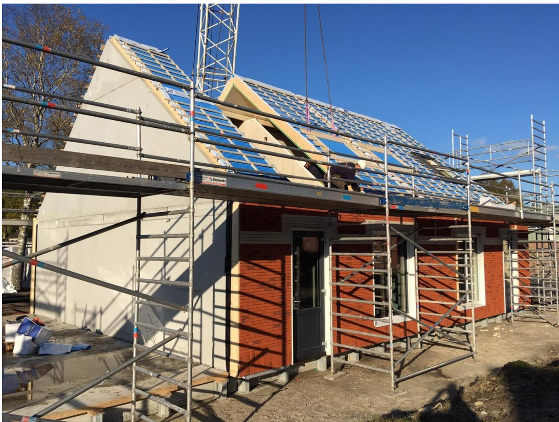
Figure 1 CMC construction as assembled and constructed on-site by BGDD
