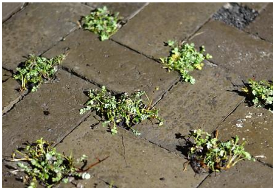
Figure 3 Bricks made from dredged sediment made by the Dutch company Waterweg. These bricks are made from local dredged sediment and let rainwater pass through to alleviate sewer systems during rain showers. Source: Waterweg Rotterdam B.V.
