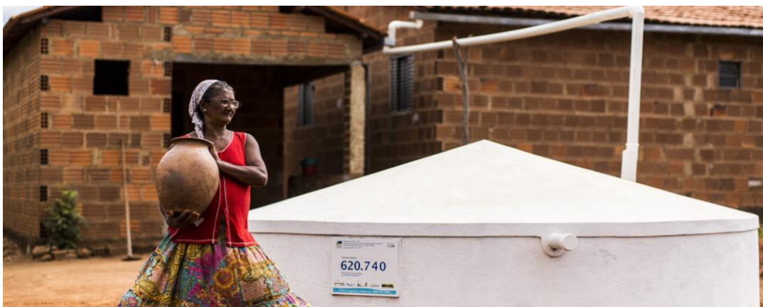
Figure 6: Individual 16.000 Liter cistern built in the Semi-arid region for securing water supply and storage during drought periods (image source: ASA, n.d.).
