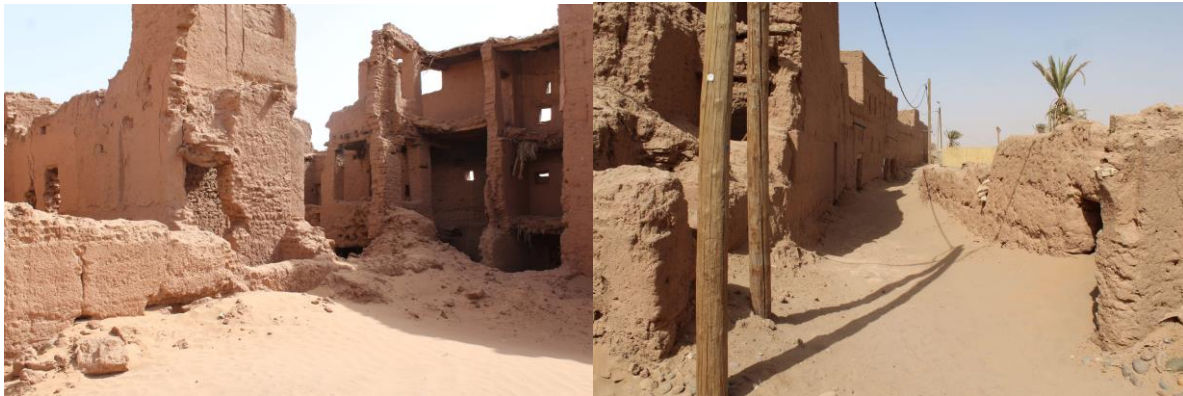
Image 27: Collapsed houses in Bounou, May 15, 2022; Image 28: Sand in front of local homes Bounou, May 15, 2022.
