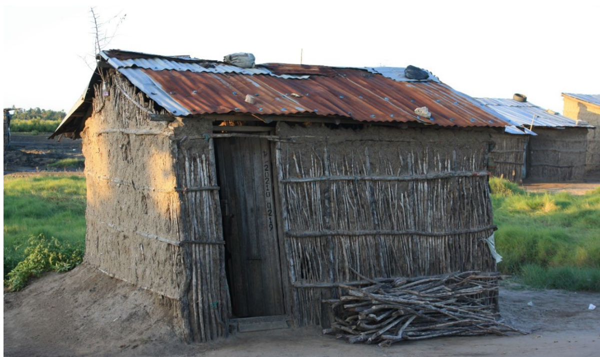
Figure 20, House constructed with mangrove wood in Icidua.
