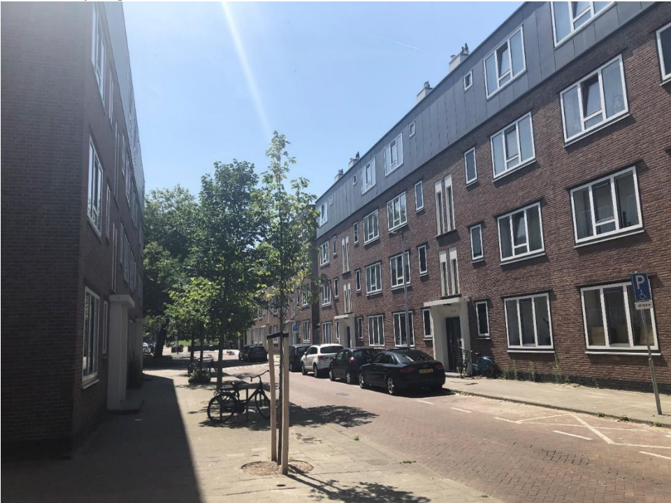
Figure 12 Street in Spangen
