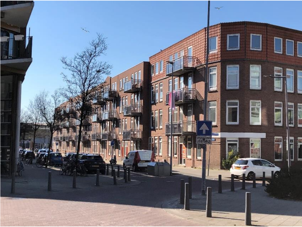
Figure 6 Street in Spangen.
