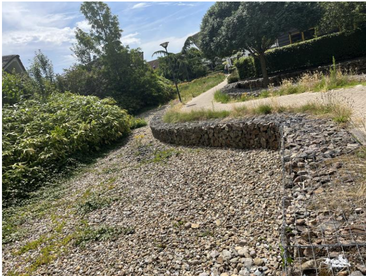
Figure 10 Wadi (or retention gravel filter pond) in De Landerijen
