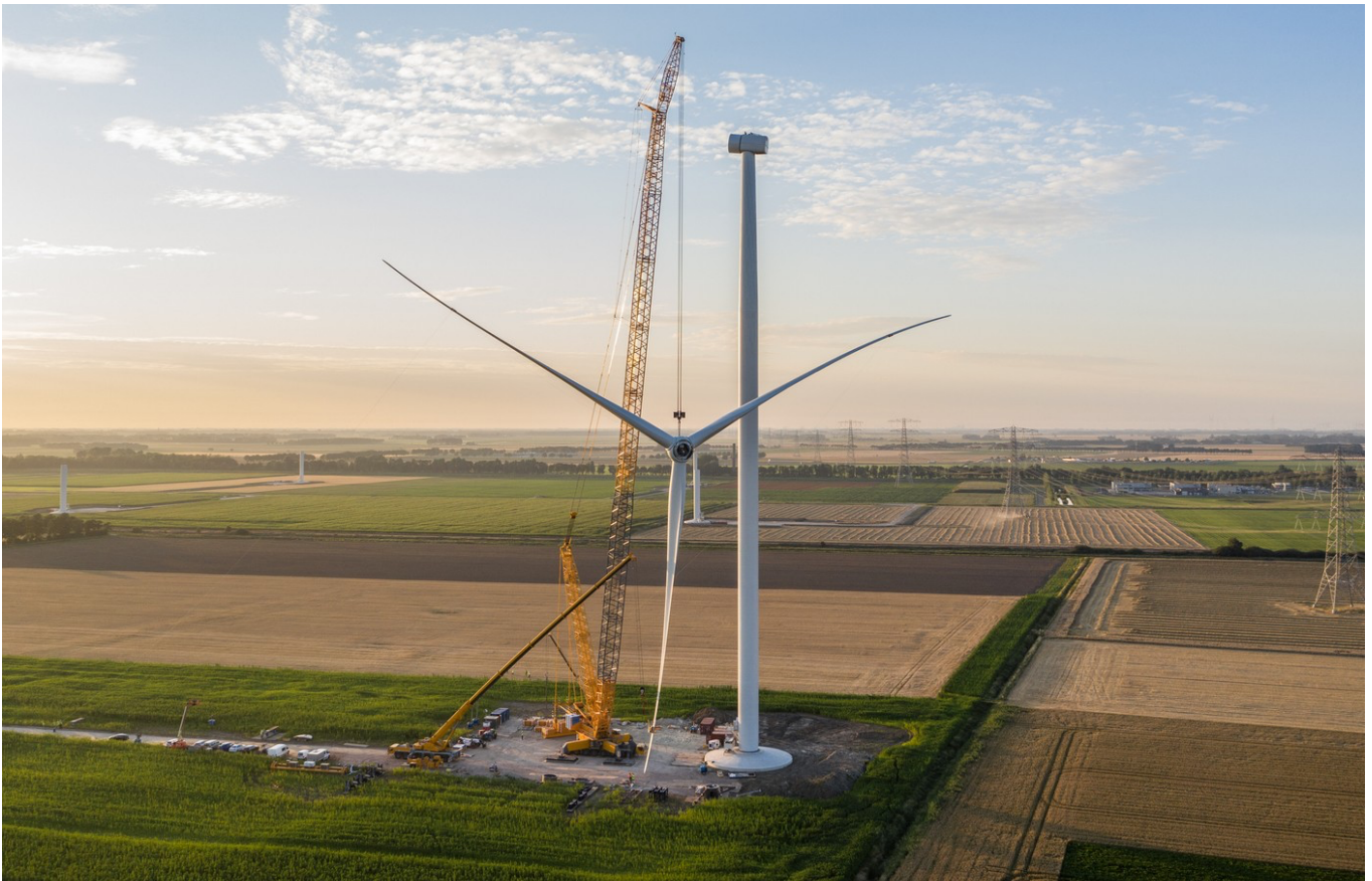
Construction of wind turbine, N33 Source: De Groene Amsterdammer
