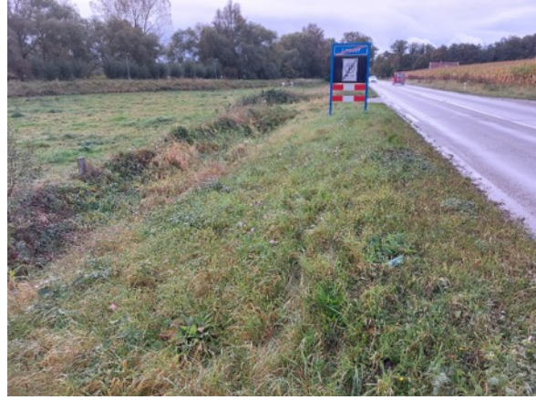
Figure E.1.14: Roadside with ditch of about 1 m deep (location 2.)
