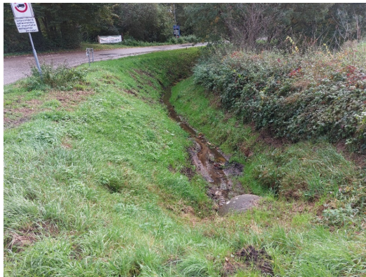
Figure 20: Deep ditch at location 15.
