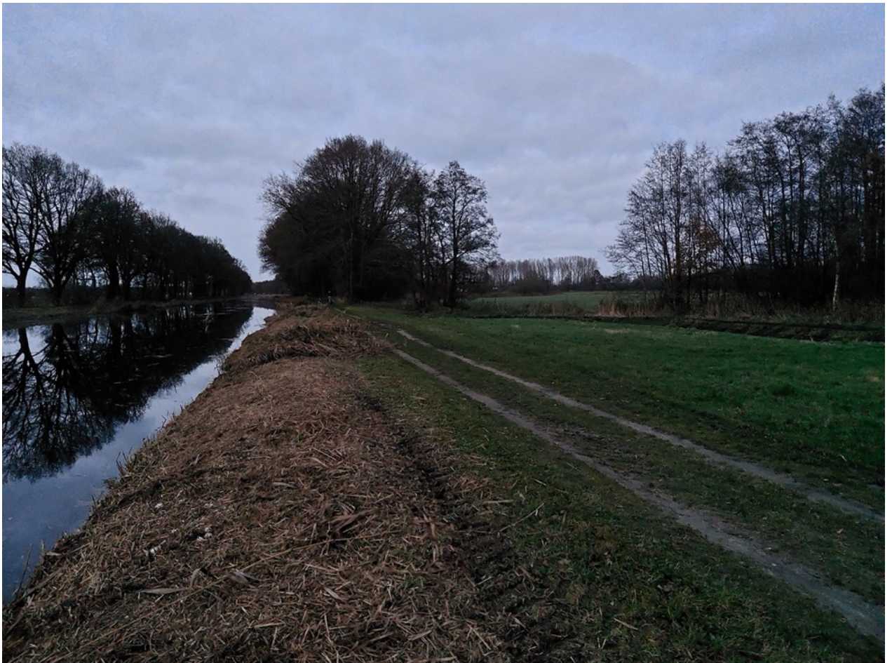
Figure D.2.32: Channel (location 16) along border of the area (visible on the far right of the picture), water surface seems to be higher than ground level of the area.
