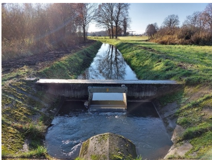
Figure D.2.14: Deep, fast-flowing ditch at location 1.
