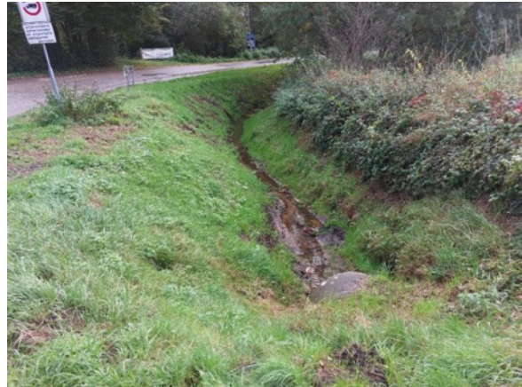
Figure E.1.15: Ditch of about 2.5 m deep, flowing directly into the Dinkel (location 3).
