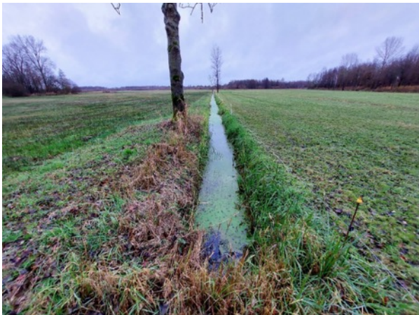
Figure D.1.18: Ditch at location 7.
