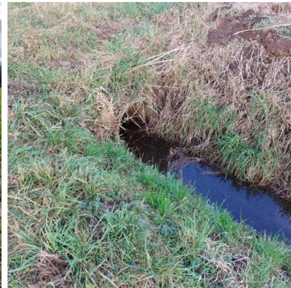
Figure E.2.14: Culvert at location 2.
