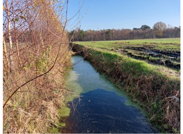
Figure C.2.18: Ditch of 1.10 m deep with 60 cm of water.
