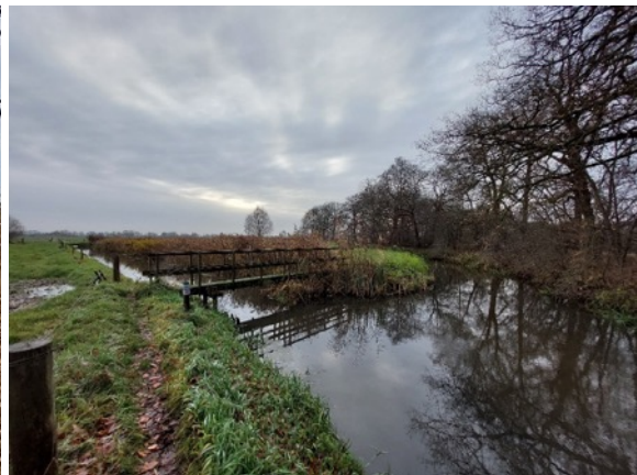
Figure D.5.15: Two flowing ditches draining the plot at location 3.
