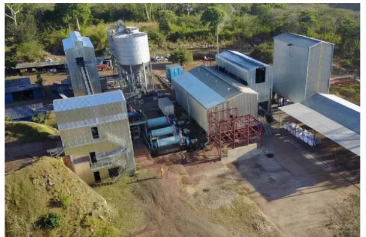
Figure 22. Aerial photo of the GK mine facilities (Mumba, 2017)
