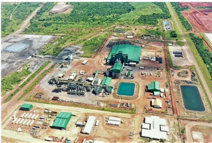
Figure 21. Aerial photo of the Syrah mine facilities (Syrah Resources, n.d.-a)
