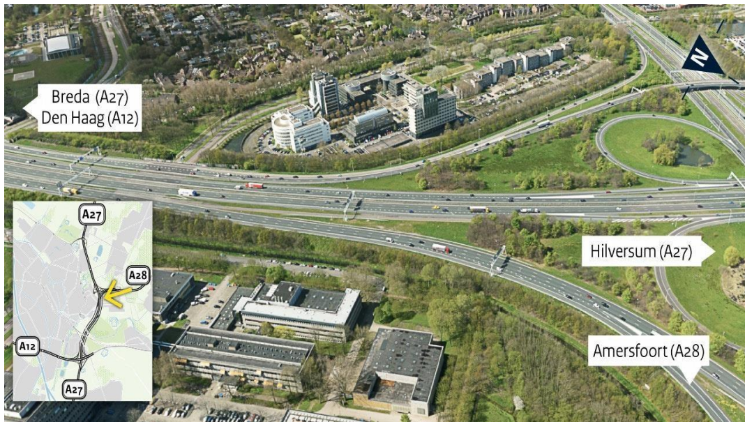
Figure 8 Current (n.d.) Retrieved from https://www.a27a12ringutrecht.nl/over+het+project/default.aspx
