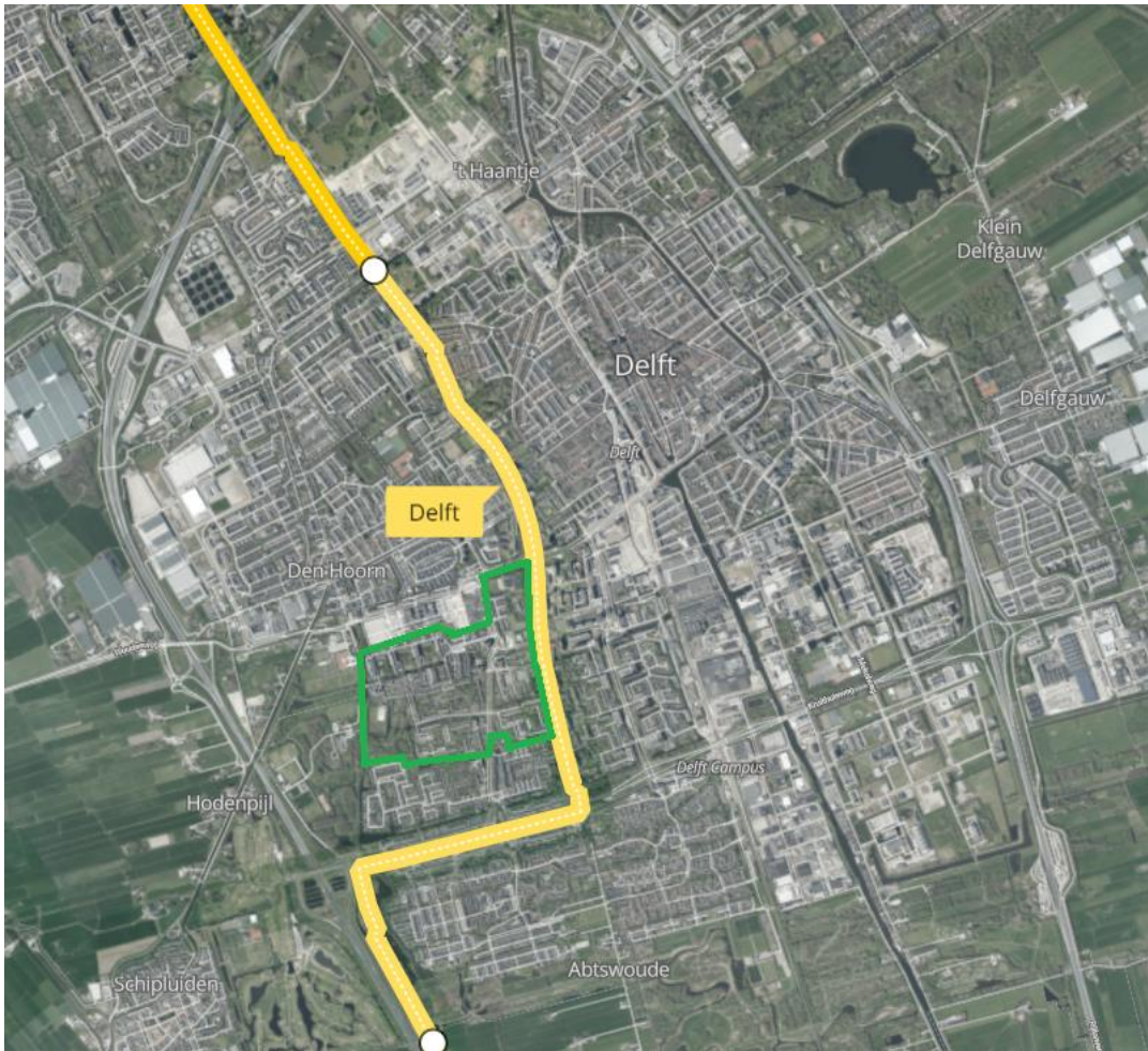
Figure 13: View of how the WarmtelinQ heat transportation pipe crosses Delft
