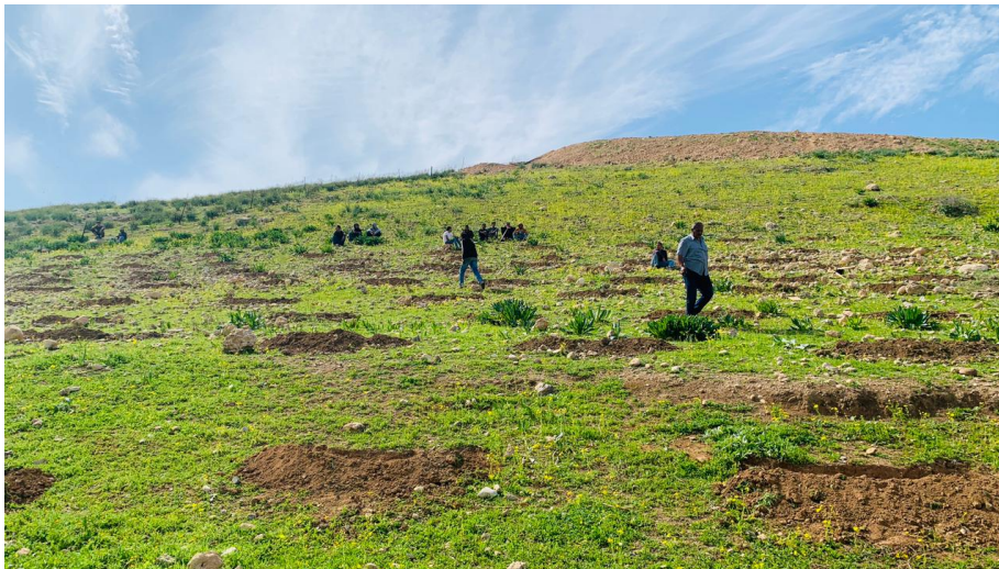
Figure 3.10: Pilot field for tree pit structures
