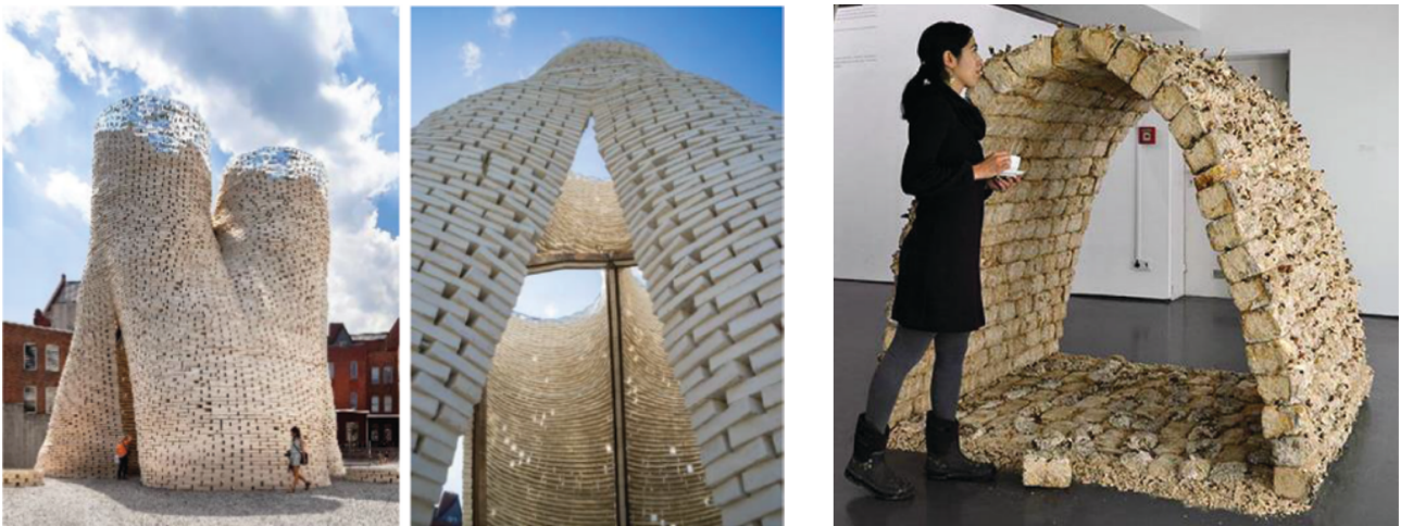
Figure 1. Examples of mycelium-based construction materials. (A) Hy-fi organic compostable tower (left image: LafargeHolcim Foundation; right image: krisgraves). (B) Mycotectural Alpha teahouse (courtesy of Philip Ross). Obtained from Jones et al., 2017.
