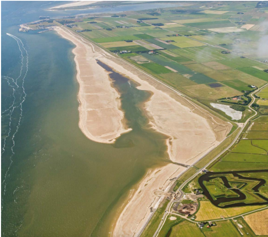
Figure 1: Aerial photo of the Prins Hendrik Sand dyke (Knaeps et al., 2019)
