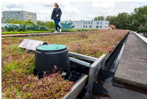
Figure 17: Green roof with Polder Roof (MetroPolder).
