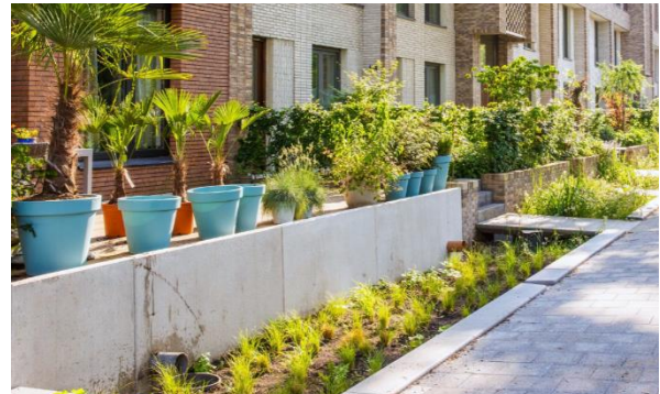
Figure 4: A new stormwater planter in Amsterdam, the Netherlands fits between the sidewalk and the housing blocks in the dense area of Zuidas (Amsterdam Zuidas).
