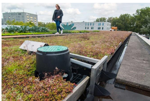
Figure 9: The first Polder Roof just after completion in 2013 (Merlijn Michon).
