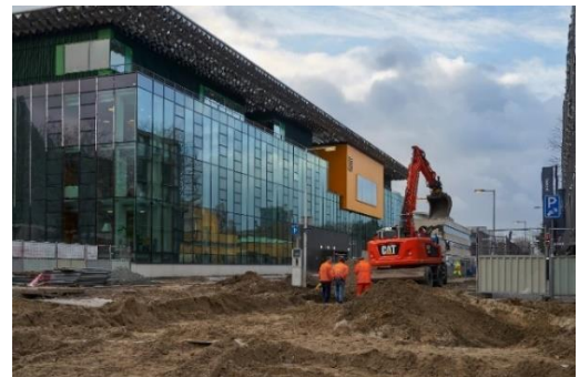
Figure 15: Project under construction January 2019 (Marcel Steinbach).
