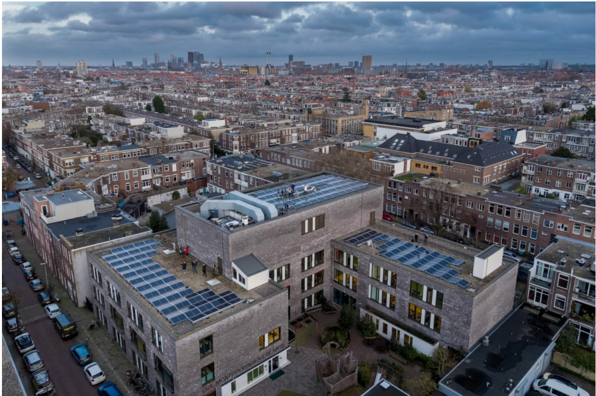
240 solar panels on the elementary schools Valkenbos and CMS Abeel (Duurzaam Den Haag, 2021)
