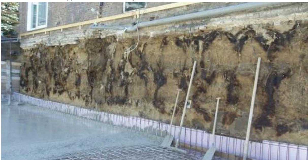
Figure 2.1.3. An injected soil underlying an existing foundation (B&P Bodeminjectie, 2012b).
