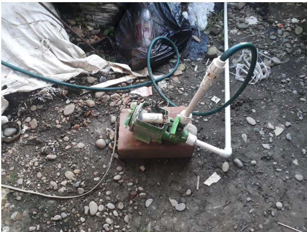
Figure 7: Resident’s extension of the water infrastructure in a low-income neighbourhood in Buenaventura, Colombia (IHE Delft, 2020).
