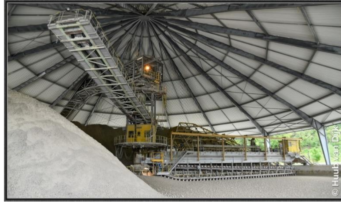
Figure 24: Raw meal storage of the Dutch cement plant in Maastricht (van Dijk, 2018).
