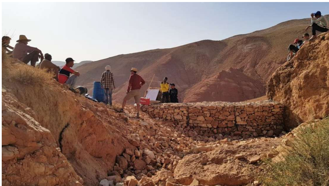
Figure 3: Villagers learning how to build gabions to slow down runoff and minimize land erosion. Retrieved from Perma-atlas.com (2021).
