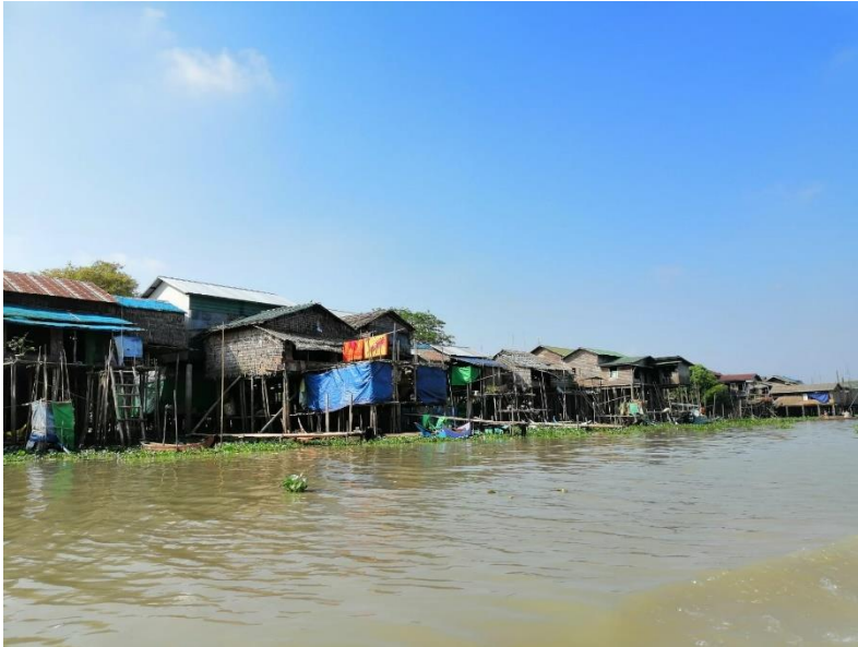
Image 6: Houses are directly situated near the stream in Hpa Yar Ni.
