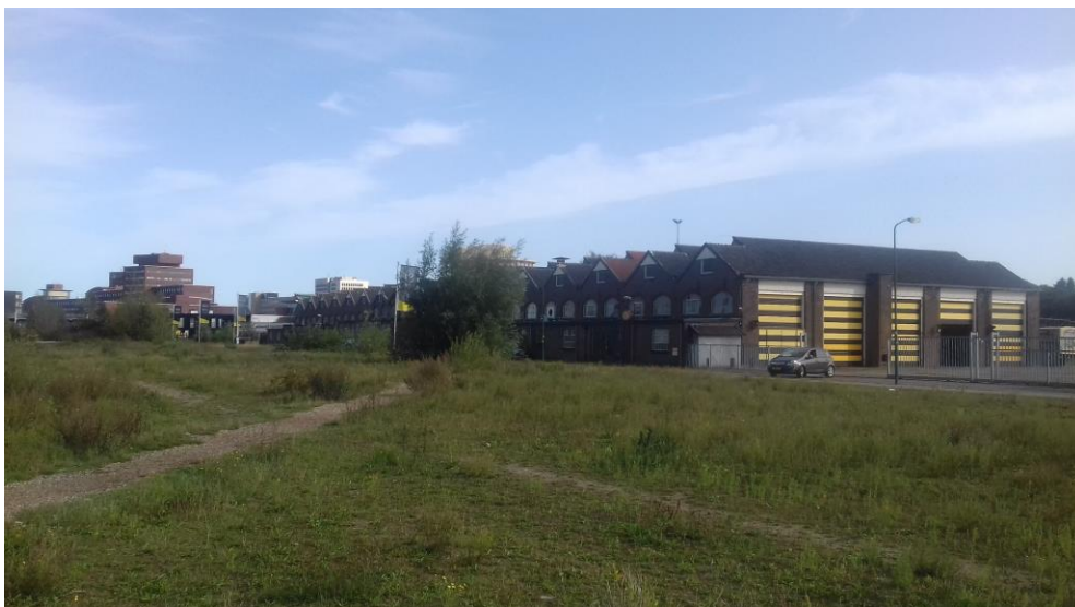
The carriage shed 'Rijtuigenloods', nowadays a national monument (Endstra, 2020)
