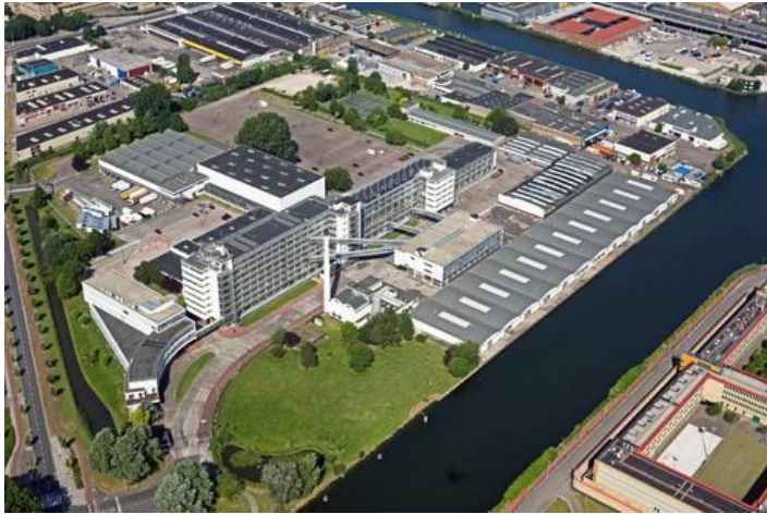
Aerial view of the Van Nelle Complex (Keuzenkamp, 2008)
