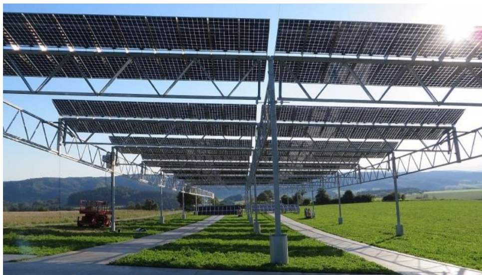
Figure 5: An example of the previous mentioned static agrivoltaic system at a height of 5m (The Vallourec Industry Magazine, 2016)
