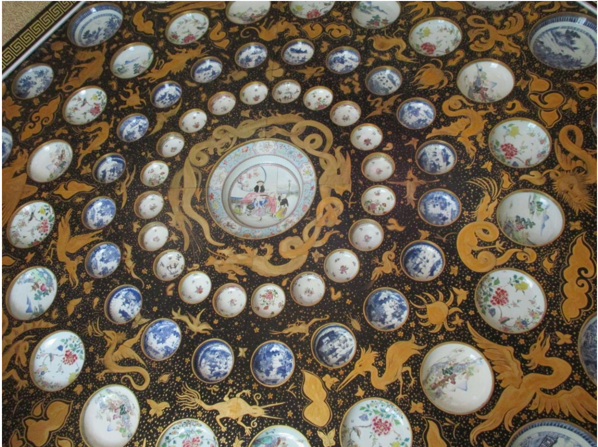
Fig. 60 – The ceiling in the tower chamber at Heeswijk Castle © Johannes Janssen.
