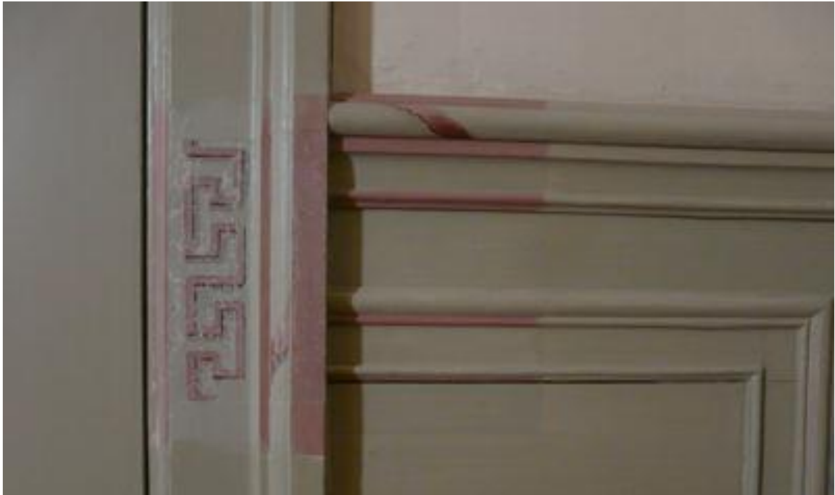
Fig. 39 – Salon 1.6, detail of reconstructed painted meander motif on doorframes and paneling © Monique Staal.
