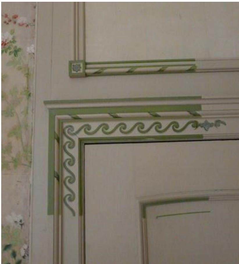
Fig. 40 - Salon 1.5, detail of reconstructed painted meander motifs on doorframes © Monique Staal.
