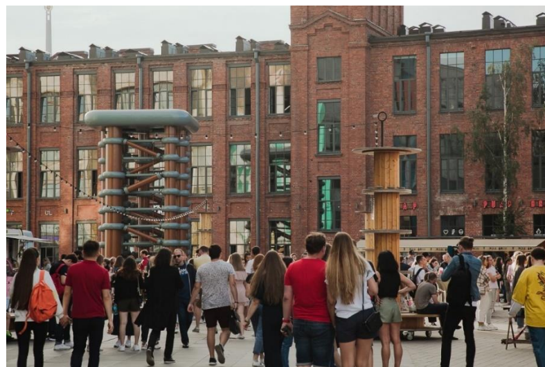
Figure 38. The research institute building 40E in 2020 (Sevkabel Port, 2020)
