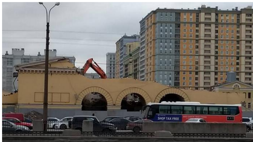
Figure 14. Demolition of the Petmol plant building, 2019. Source: https://moika78.ru/news/2019-03-23/207837-na-moskovskom-snosyat-zdaniya-petmola/
