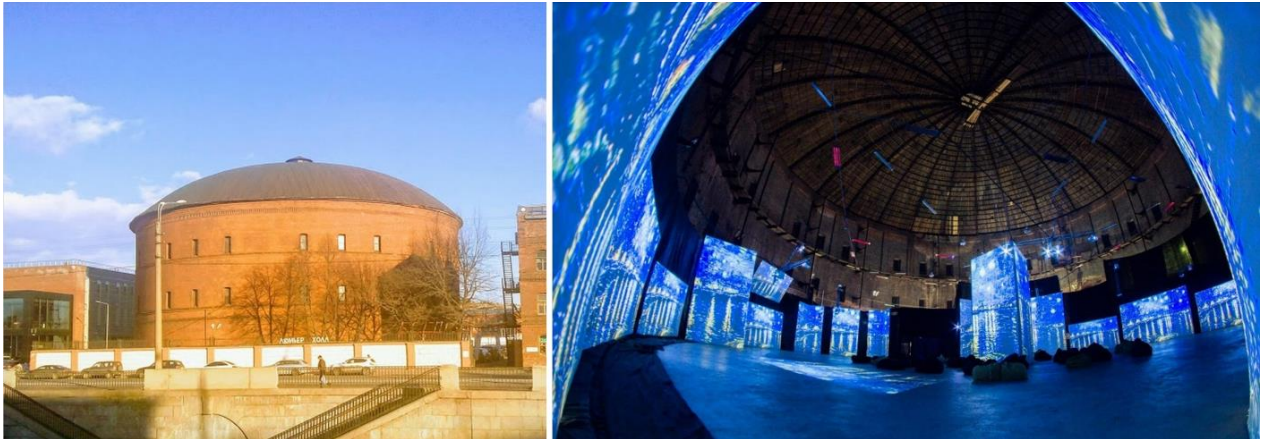
Figure 20. Gasholder Building – New Planetarium (Organisation of World Heritage Cities, 2019)
