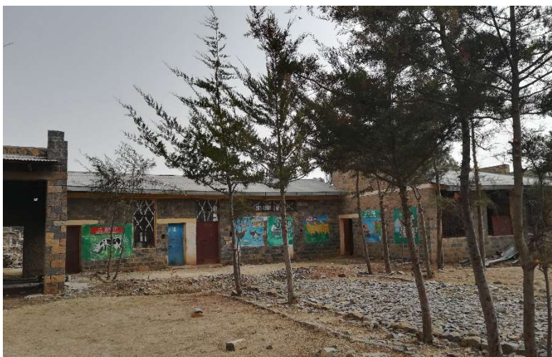
Figure 6.1. The exterior of the extension office in Mere-Mieti (v).
