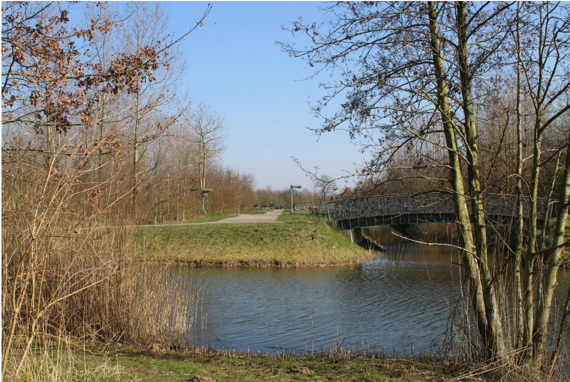
Figure B.5 Bridge (T. Sneijder)
