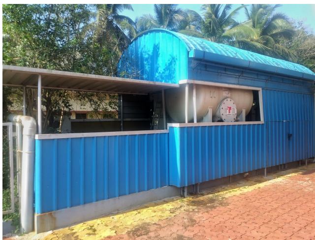
Picture 20: A decentralised water treatment plant on the premise of an apartment building in Udupi. The water that exits the building runs through this installation in order to clean it up to water effluent standards so that it can be released into the environment.
