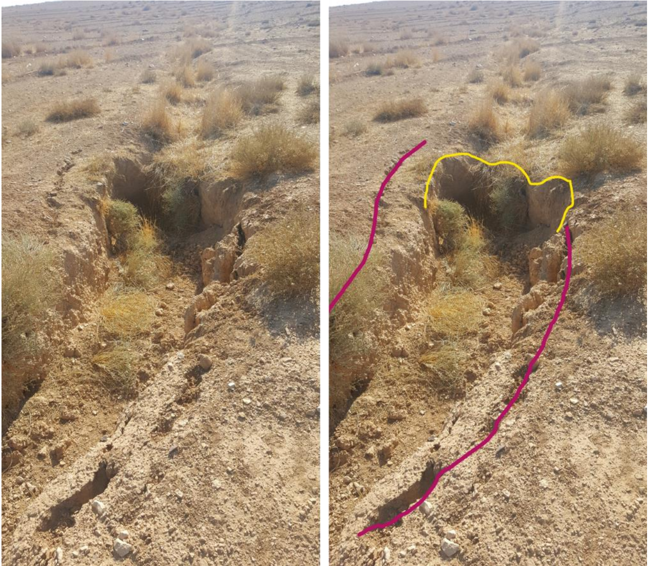
Figure 40: The starting point of the gully and headward erosion as observed in the field. Undercutting takes place at the yellow line, the purple line depicts spliced earth.
