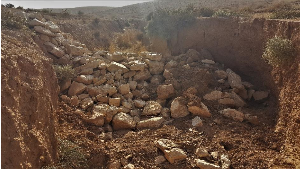
Figure 49: Failed gully plug located in the treated watershed. Increased erosion was seen on the right where the side bank collapsed.
