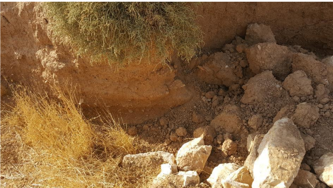
Figure 45: Vegetation holding soil together while the side collapses.
