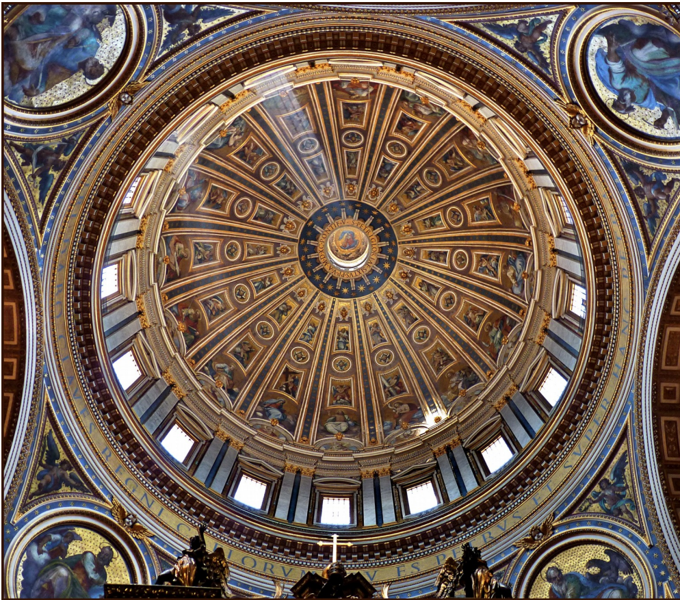
Figure 11. Interior of the dome of the St. Peter's Basilica. Cavalier d'Arpino, ca 1620, Rome.
