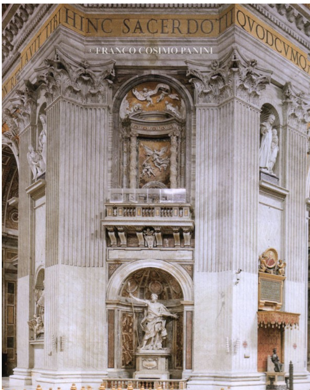
Figure 5. Southwestern pier of the dome. Donato Bramante, ca 1506-1514, Rome. The Solomonic columns can be seen above the loggia.
