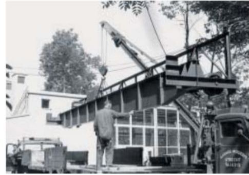
Figure 29: The construction of a new laboratory hall at FOM-Rijnhuizen. Photo archives DIFFER.
