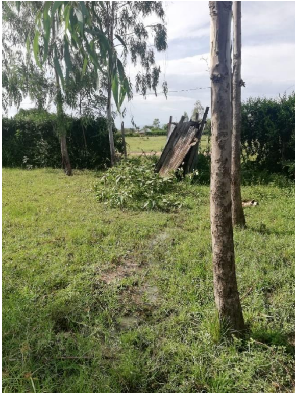
Photo 4 - Collapsed latrine in flood-prone sub-county Nyakach. Author's own.
