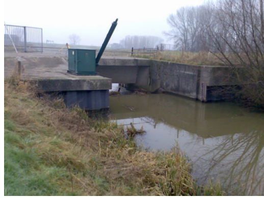
(b) Weir 103HOE, viewed from the upper part of the weir.
