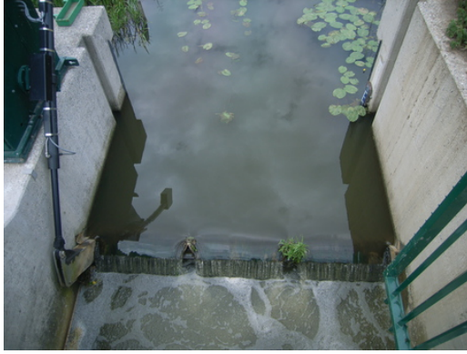
(a) Weir 102BFS, viewed from the lower part of the weir.
