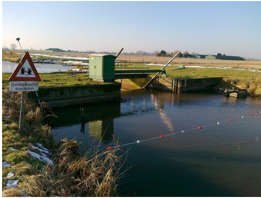
(c) Weir 104OYE, viewed from the upper part of the weir.
