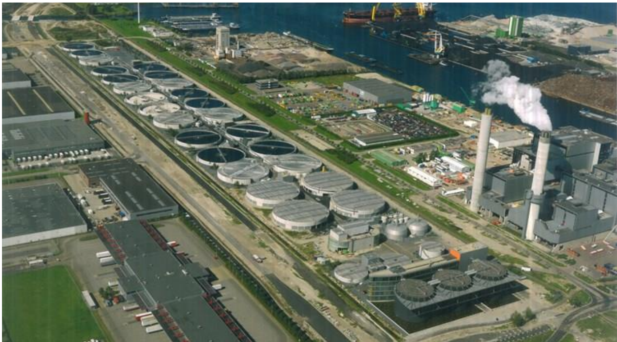
FIGURE 3: OVERVIEW OF THE WWTP AMSTERDAM WEST (WATERNET, 2019)
